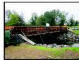
Broadway Ave. Bridge
