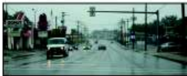
Cleveland Ave. Repaving
