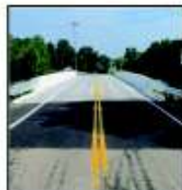
Kemaury Ave. Bridge
